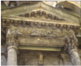
ravenswood ivanhoe detail of stonework
