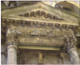
ravenswood ivanhoe detail of stonework
