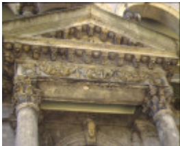
ravenswood ivanhoe detail of stonework
