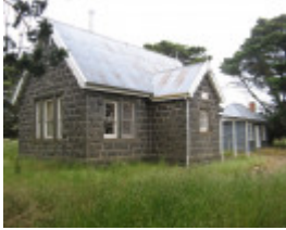
Former Leigh Shire Hall and toll house
