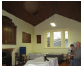
Former Leigh Shire Hall interior
