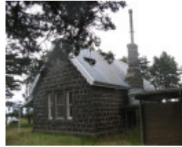
Former Leigh Shire Hall rear view
