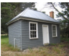
Former Leigh Shire Hall former Hesse toll house
