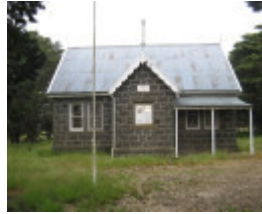
Former Leigh Shire Hall
