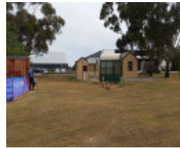
Context showing Harricks Cottage with the demounted prefabricated building under the tarpaulin May 2018
