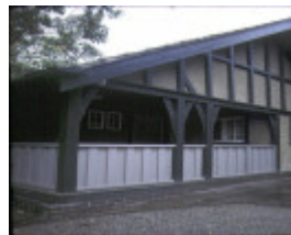
Waller house detail of front verandah
