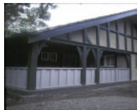
Waller house detail of front verandah
