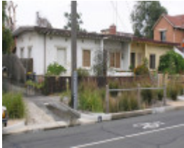
EXPERIMENTAL CONCRETE HOUSES SOHO 2008
