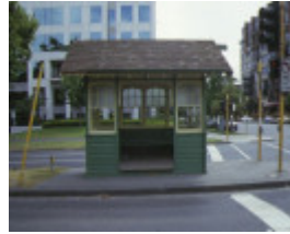
1 tram shelter cnr st kilda rd and lorne st melbourne east elevation dec1999
