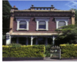
1 residence jolimont terrace jolimont front elevation nov1980
