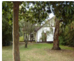
h00054 croydon maternal health centre may05 north side3
