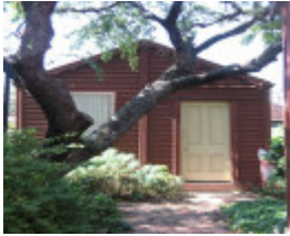
BELLHOUSE IRON HOUSE SOHE 2008
