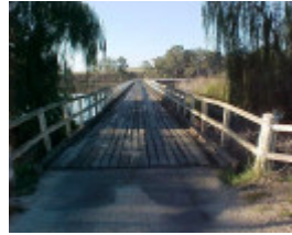
1 kirwans bridge bailieston
