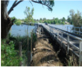
KIRWANS BRIDGE SOHE 2008
