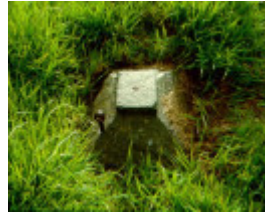
1 south base stone coverstone intact june01
