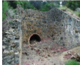
WALKERVILLE LIME KILNS SOHE 2008
