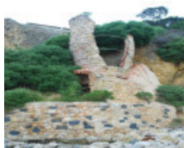
WALKERVILLE LIME KILNS SOHE 2008
