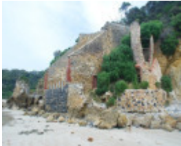
WALKERVILLE LIME KILNS SOHE 2008
