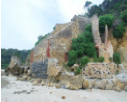
WALKERVILLE LIME KILNS SOHE 2008
