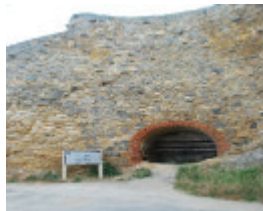
WALKERVILLE LIME KILNS SOHE 2008
