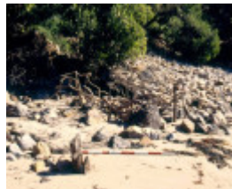
h02043 walkerville jetty timbers 2003
