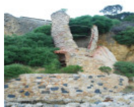
WALKERVILLE LIME KILNS SOHE 2008
