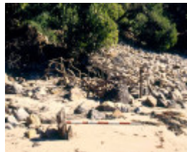
h02043 walkerville jetty timbers 2003
