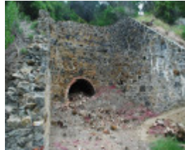
WALKERVILLE LIME KILNS SOHE 2008
