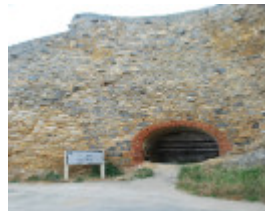
WALKERVILLE LIME KILNS SOHE 2008
