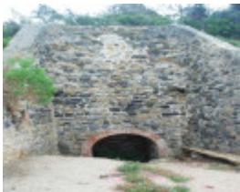
WALKERVILLE LIME KILNS SOHE 2008
