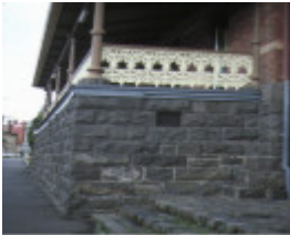
former police station ballarat detail of verandah
