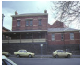
former police station ballarat rear view
