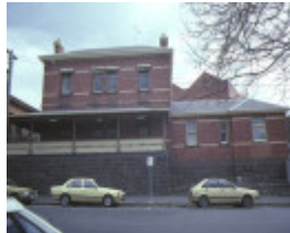
former police station ballarat rear view
