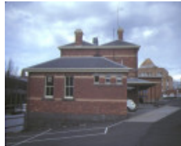
former police station ballarat side elevation
