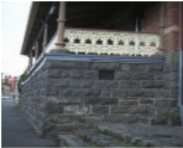
former police station ballarat detail of verandah
