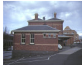
former police station ballarat side elevation
