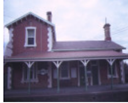
1 kangaroo flat railway station complex front elevation jul1984
