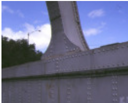
iron bridge maribyrnong river detail of iron siding
