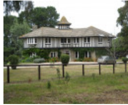
Westerfield from north
