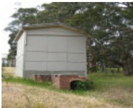
Westerfield_drying shed & furnace_KJ_Dec 08
