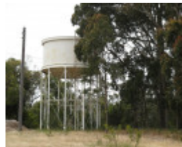
Westerfield_Frankston_elevate water tank_KJ_Dec 08
