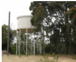
Westerfield_Frankston_elevated water tank_KJ_Dec 08
