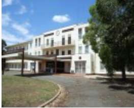
FORMER MILDURA BASE HOSPITAL SOHE 2008
