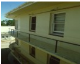
Former Mildura Base Hospital West Wing 2001
