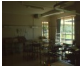
Former Mildura Base Hospital Ground Floor 2001
