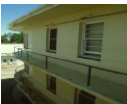
Former Mildura Base Hospital West Wing 2001
