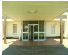
Former Mildura Base Hospital Porte Cochere 2001
