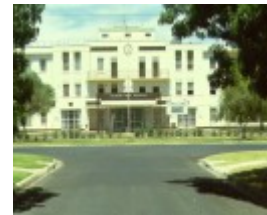
Former Mildura Base Hospital Main Entrance 2001
