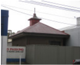
City of Brunswick Electricity Supply transformer station (former) - 188 Brunswick Road, Brunswick
