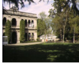
1 ross house kew view of arched verandah front
