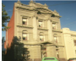
1 ballarat trades hall camp street ballarat front elevation
