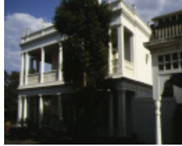
1 studley house kew front view
