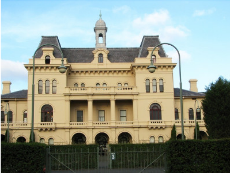
FORMER WILLSMERE HOSPITAL SOHE 2008
