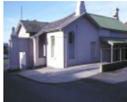
former willsmere hospital kew gatehouse june 1988
