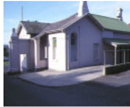
former willsmere hospital kew gatehouse june 1988
