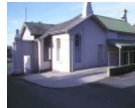
former willsmere hospital kew gatehouse june 1988
