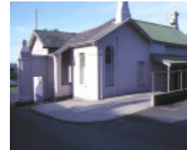
former willsmere hospital kew gatehouse june 1988
