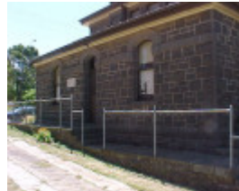
H01471 kilmore court house exterior side april 2003
