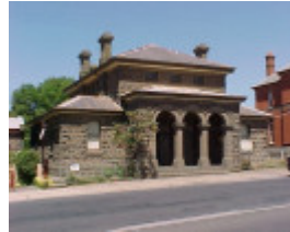
H01471 1 kilmore court house exterior april 2003
