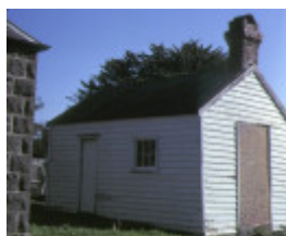
1 whitburgh cottage piper street kilmore outbuilding
