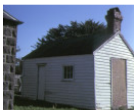
1 whitburgh cottage piper street kilmore outbuilding
