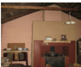
Interior - outbuilding east wing. Aug 2007.
