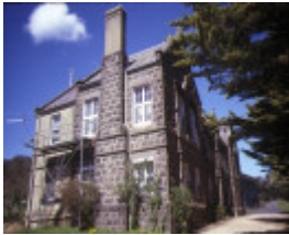
kilmore district hospital rutledge street kilmore side elevation oct1985
