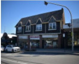
Front facade of the Shop facing High Street
