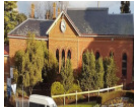
Cranbourne Shire Offices Public Hal Court House and Post Office Complex - view from intersection of South Gippsland Hwy
