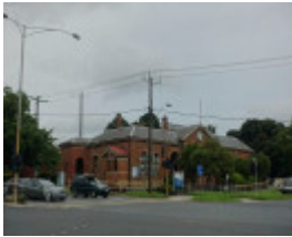
Cranbourne Shire Offices Public Hal Court House and Post Office Complex - view from intersection of South Gippsland Hwy and Sladen Street
