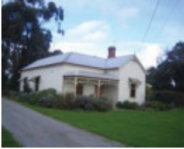
10 Ballarto Road - north east view
