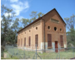
BILLABONG PUMPING STATION SOHE 2008
