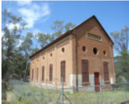
BILLABONG PUMPING STATION SOHE 2008
