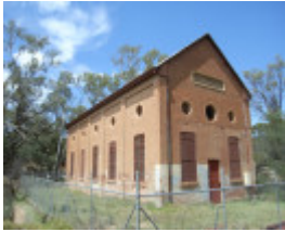
BILLABONG PUMPING STATION SOHE 2008
