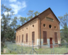
BILLABONG PUMPING STATION SOHE 2008
