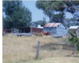
Fernlea - former dairy and machinery sheds
