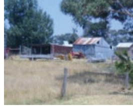
Fernlea - former dairy and machinery sheds
