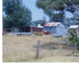
Fernlea - former dairy and machinery sheds
