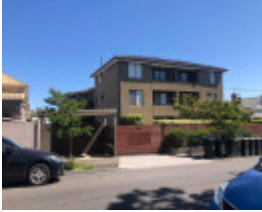
11-13 Llaneast Street, Armadale
