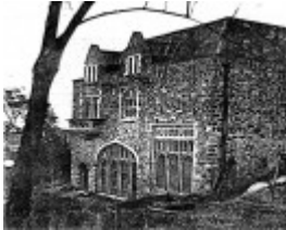
133 - Montsalvat Hillcrest Ave Eltham - Main (south) Facade of the Great Hall, photographed in 1949? - NOTE the secondhand windows, slate roof and the local stone walls - Shire of Eltham Heritage Study 1992
