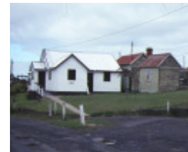
korumburra railway station complex station street korumburra outbuildings may1984
