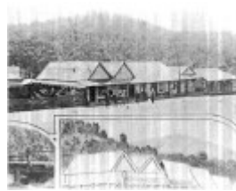
166 - St Andrews Hotel Palm KangGround St Andrews Rd 02 - 'The Leader', 2 November, 1929 - the existing hotel and adjacent shop buildings are clearly evident in this photograph - NOTE the young Canary Island Palm tree (ELHPC NO.163) - Shire of Eltham Heri
