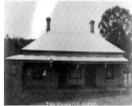
166 - St Andrews Hotel Palm KangGround St Andrews Rd 05 - Demolished Research Hotel - A very different hotel building constructed all at one time (ELHPC NO.502.) - Shire of Eltham Heritage Study 1992
