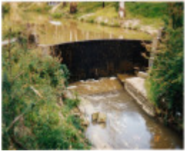
Smith Dam Karingal Drive Eltham Colour 1 - Shire of Eltham Heritage Study 1992
