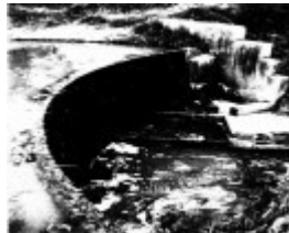
175 - Smith Dam Karingal Drive Eltham 02 - Shire of Eltham Heritage Study 1992
