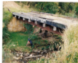
Smith Dam Karingal Drive Eltham Colour 2 - Shire of Eltham Heritage Study 1992
