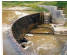
Smith Dam Karingal Drive Eltham Colour 3 - Shire of Eltham Heritage Study 1992
