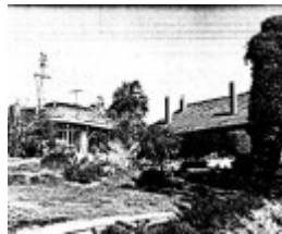
184 - Old Brinkkoter House 32 Lindon Strike Ct 03 - Shire of Eltham Heritage Study 1992
