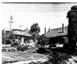
184 - Old Brinkkotter House 32 Lindon Strike Ct 03 - Shire of Eltham Heritage Study 1992
