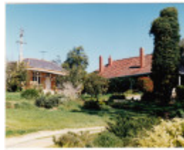
Old Brinkkoter House 32 Lindon Strike Ct Colour 2 - Shire of Eltham Heritage Study 1992
