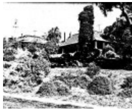
184 - Old Brinkkoter House 32 Lindon Strike Ct 02 - Shire of Eltham Heritage Study 1992
