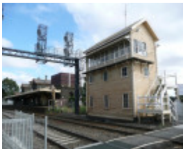
KYNETON RAILWAY STATION COMPLEX SOHE 2008
