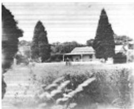
192 - Wingrove Cottage Pines 672 674 Main Rd - Old photograph (ELHPC no?) - Shire of Eltham Heritage Study 1992
