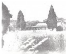
Wingrove Cottage Pines 672 674 Main Rd Black & White 1 - Shire of Eltham Heritage Study 1992
