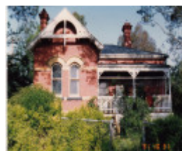
State School 209 Residence Pines 690 Main Rd Colour 2 - Shire of Eltham Heritage Study 1992
