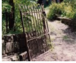
Jarrold Cottage Shop Studio 701 Main Rd Colour 3 - Shire of Eltham Heritage Study 1992
