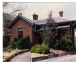
Former Police Complex 728 Main Rd Eltham Colour 1 - Shire of Eltham Heritage Study 1992
