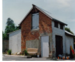
Former Police Complex 728 Main Rd Eltham Colour 3 - Shire of Eltham Heritage Study 1992
