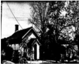
199 - Court House 730 Main Rd Eltham - Shire of Eltham Heritage Study 1992
