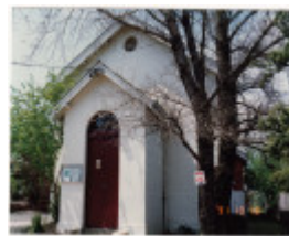
Court House 730 Main Rd Eltham Colour 1 - Shire of Eltham Heritage Study 1992
