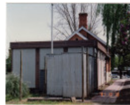
Court House 730 Main Rd Eltham Colour 2 - Shire of Eltham Heritage Study 1992
