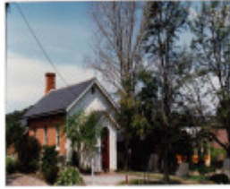
Court House 730 Main Rd Eltham Colour 5 - Shire of Eltham Heritage Study 1992
