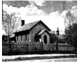
199 - Court House 730 Main Rd Eltham 02 - 1949? photograph showing the court house, previous/original timber picket fence, site planting and the police residence chimneys - Shire of Eltham Heritage Study 1992
