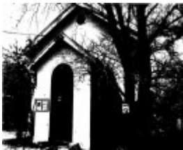
199 - Court House 730 Main Rd Eltham 04 - Shire of Eltham Heritage Study 1992
