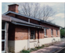
Court House 730 Main Rd Eltham Colour 3 - Shire of Eltham Heritage Study 1992
