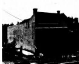
201 - Shop Dwelling 738 Main Rd Eltham - Shire of Eltham Heritage Study 1992
