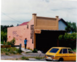
Shop Dwelling 738 Main Rd Eltham Colour - Shire of Eltham Heritage Study 1992
