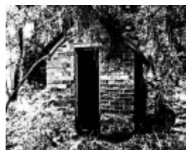
202 - Living Learning Centre 739 Main Rd Eltham 04 - Shire of Eltham Heritage Study 1992
