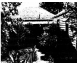
202 - Living Learning Centre 739 Main Rd Eltham 03 - Shire of Eltham Heritage Study 1992
