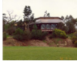
Eltham Community Centre Main Rd Eltham Colour 4 - Shire of Eltham Heritage Study 1992
