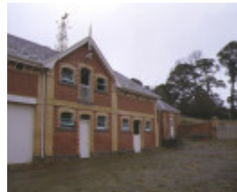
st agnes homestead calder hwy kyneton stables entrance jul1999
