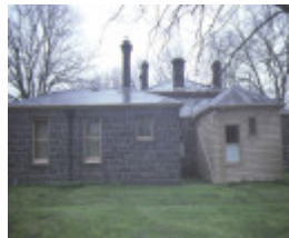
kyneton court house hutton street kyneton rear elevation sep1984
