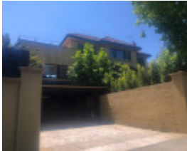
367 Dandenong Road, Armadale
