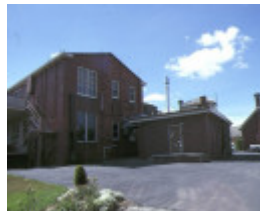
kyneton district hospital simpson street rear view
