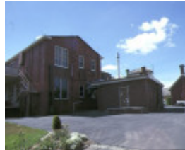
kyneton district hospital simpson street rear view
