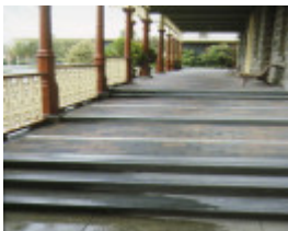
kyneton district hospital simpson street verandah oct1992
