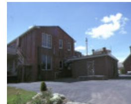
kyneton district hospital simpson street rear view
