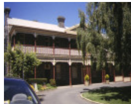
1 kyneton district hospital simpson street front view nov1997
