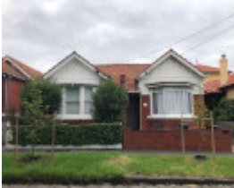
23-25 Banole Avenue, Prahran
